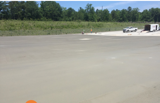
4 Close-up of CCP surface while finishing.
