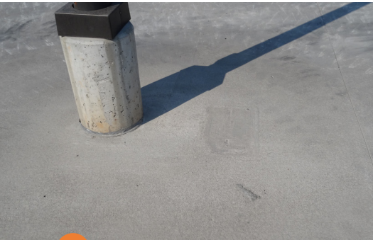
5 The ability to work CCP around structures.
