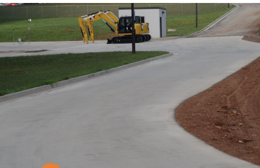
6 Completed asymmetrical installation of CCP.
