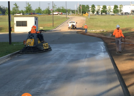
2 Freshly placed CCP around catch basin.
